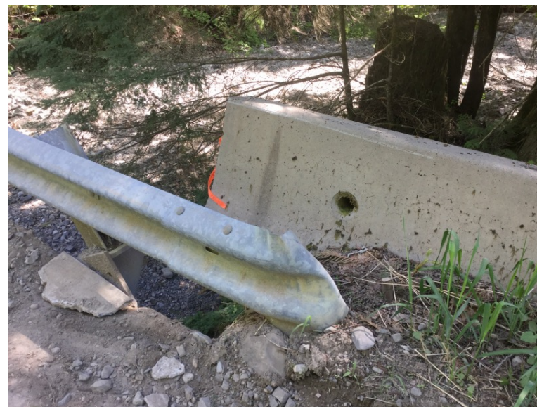
Downstream right approach barrier alignment
