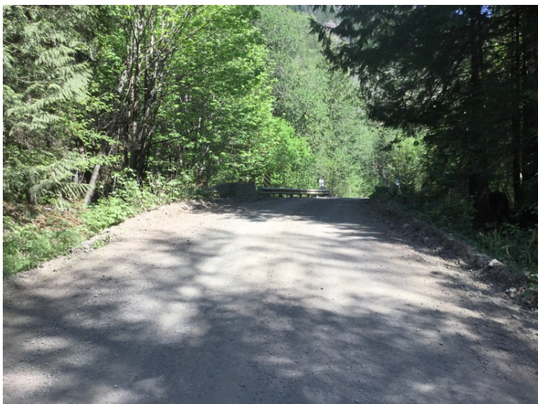
Approach from Right Bank when facing downstream
