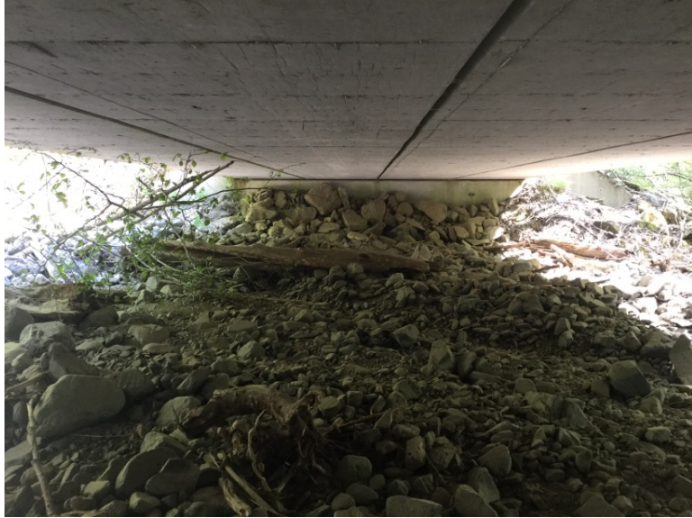
Left Bank Abutment when facing downstream
