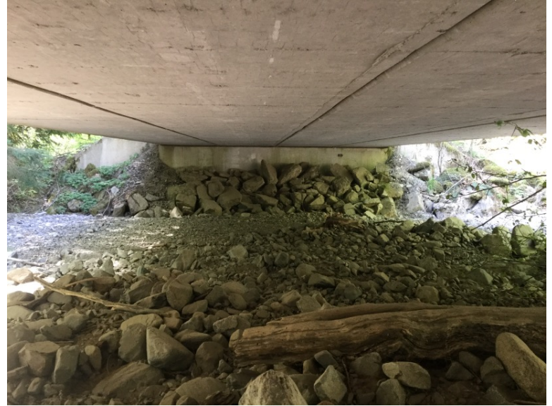
Right Bank Abutment when facing downstream
