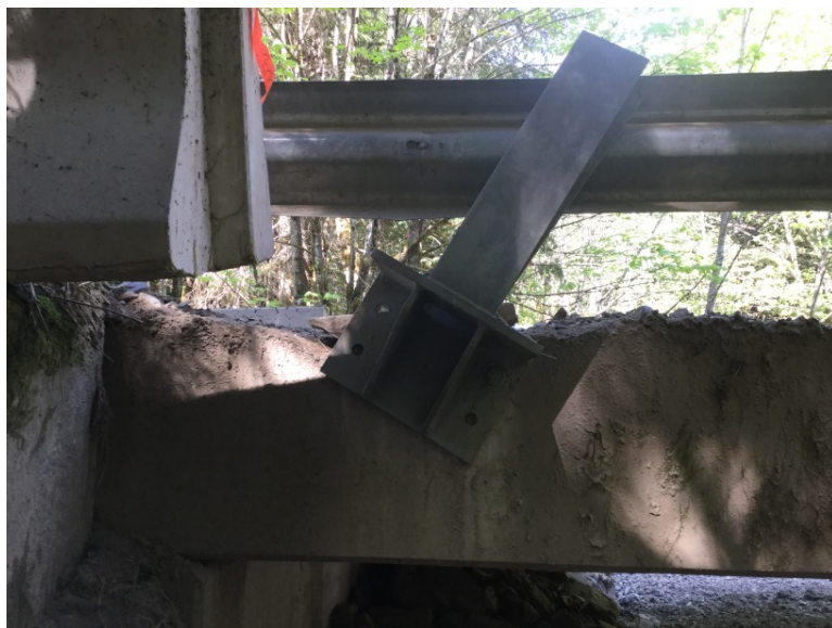
Downstream right approach steel riser condition
